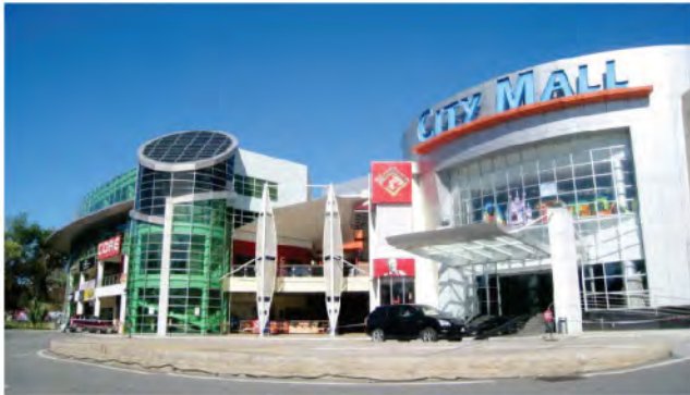
City Mall completed in 2008, developed by Pan Far Eastern Sdn Bhd
