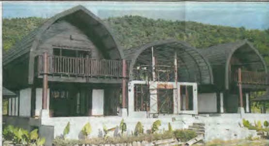
Kudat Riviera Villa build progress as at September 2013.
