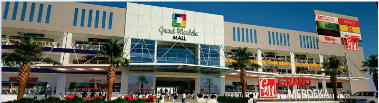
The Grand Merdeka Mall at Menggatal is currently under construction. The mall is developed by Grand Merdeka Development Sdn Bhd.
