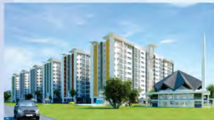
Timbok Jaya Apartment, Tuaran
