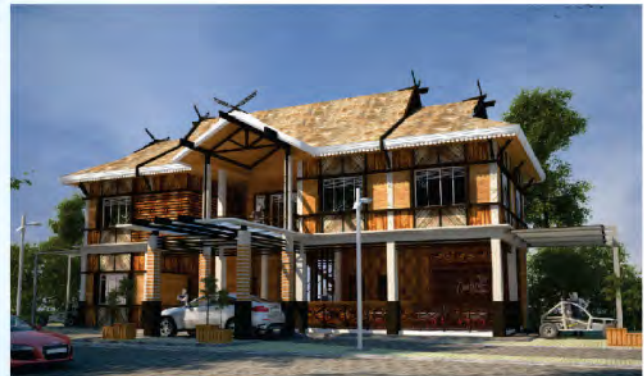
Clubhouse & Reception Building
