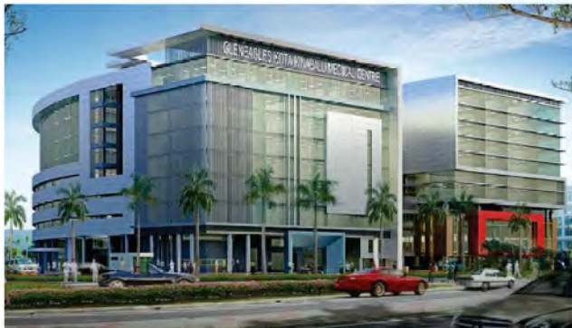
Ongoing construction, Riverson Walk is being developed by Riverson Corporation Sdn Bhd
