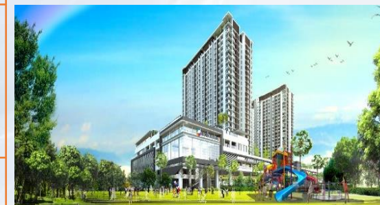
ELEMEN UTARA KK PHASE 3 TOWER A
